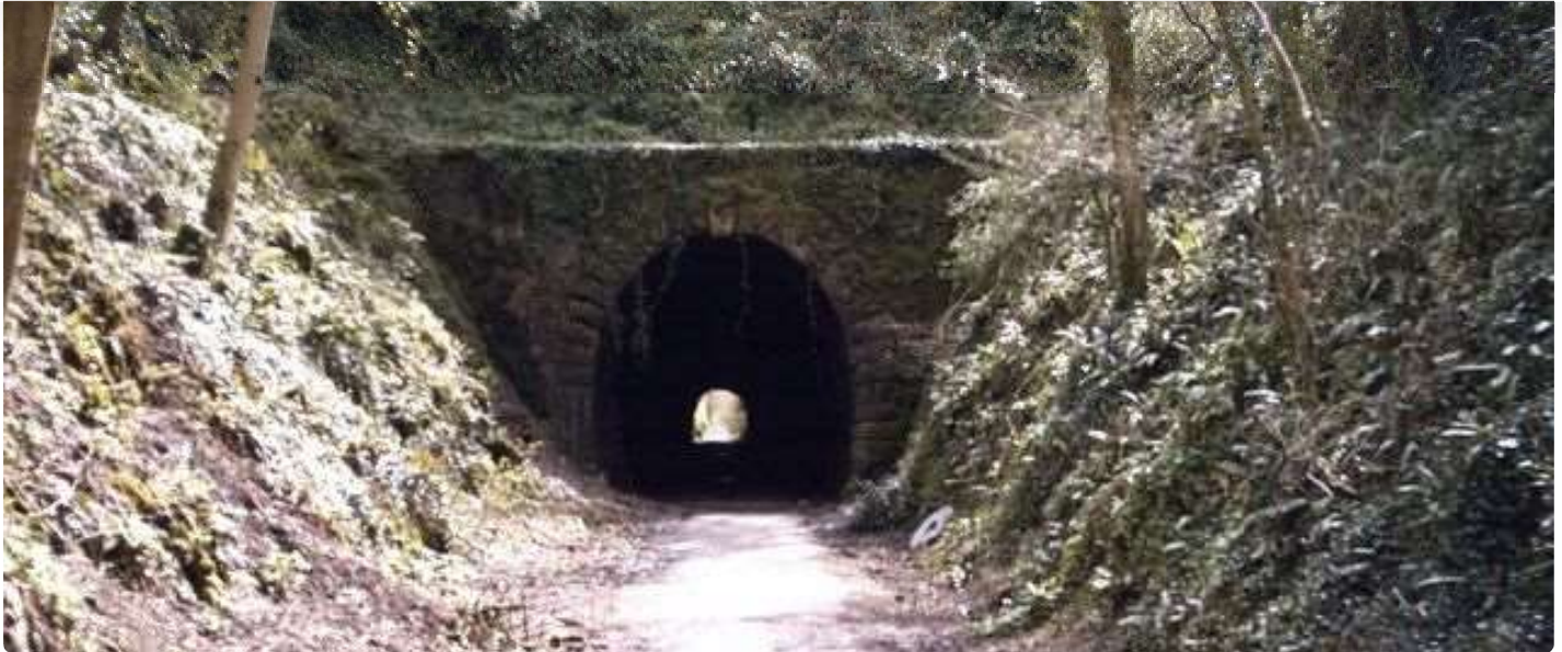
Temporary closure on the Strawberry Line at Winscombe tunnel
