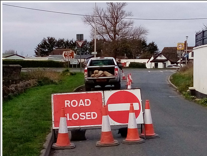
A370 Anchor Inn / Catherines Inn Junction
