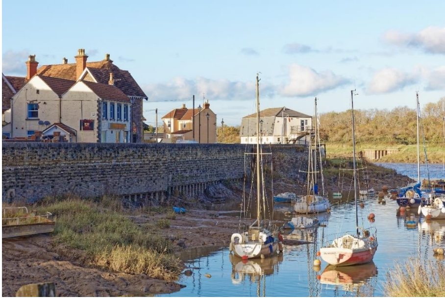
Images 5 and 6. At Pill, the walls and flood gates prevent high tides and storm surges that flow up the River Avon from flooding nearby properties.
