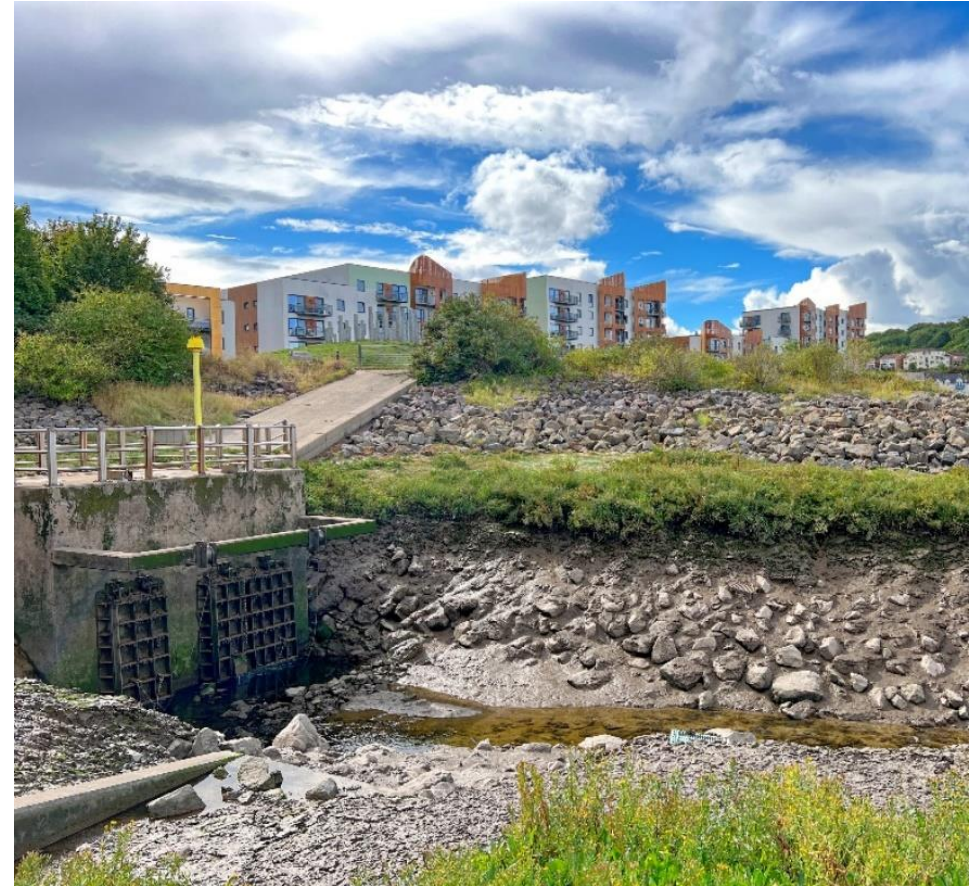
Image 12. This is a tidal flap at Portishead's end of the Portbury Ditch. The flap lets water out when the tide is low and holds the tide back when the sea rises against the flap.
