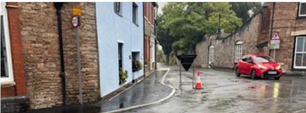
Improved footways on the way to school in Wrington
