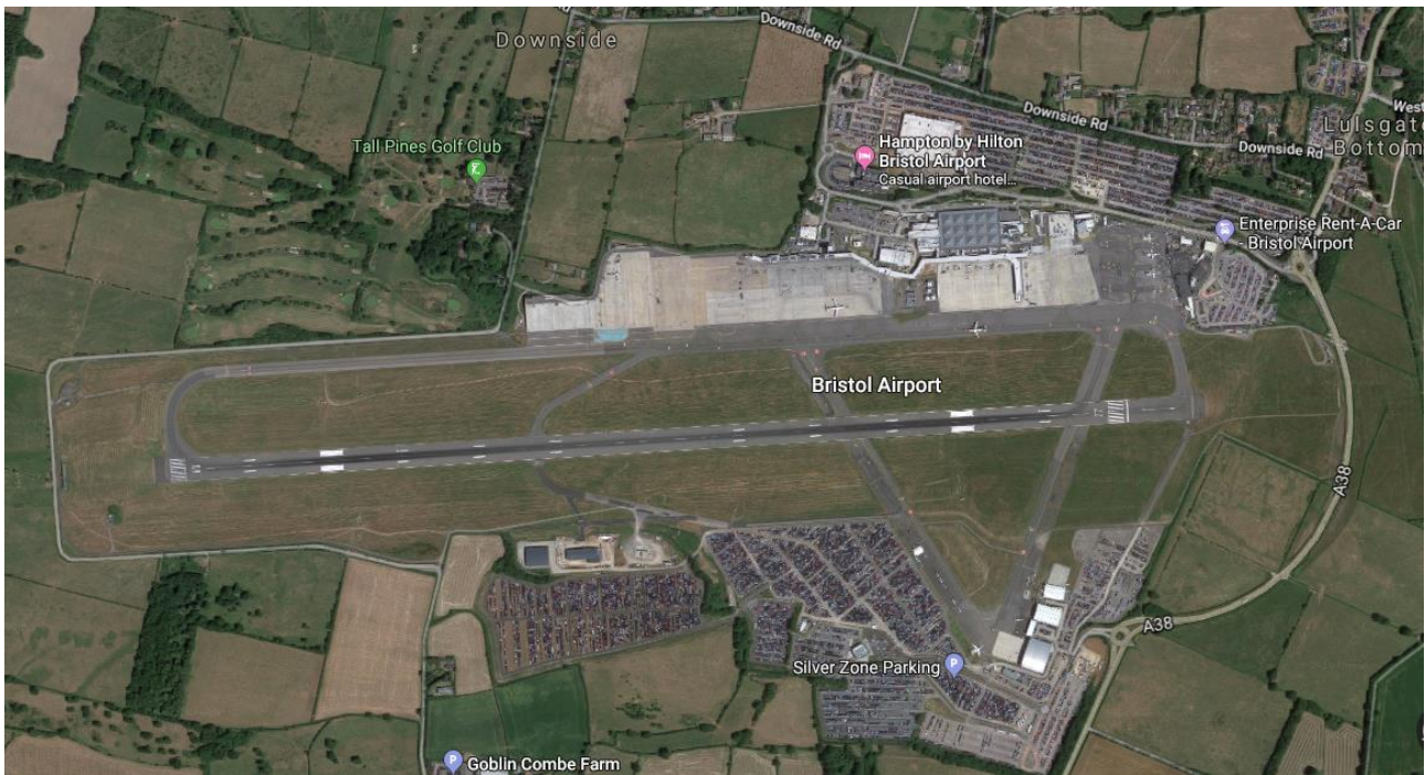
Figure B Bristol Airport Site
