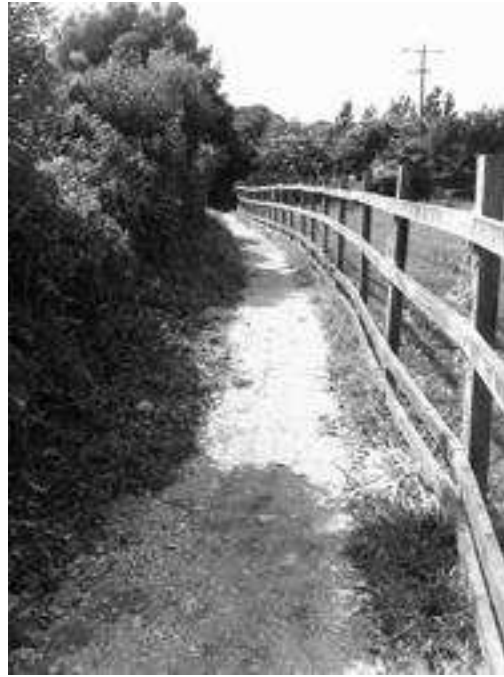
The section of newly surfaced footpath from the allotments towards Purn
