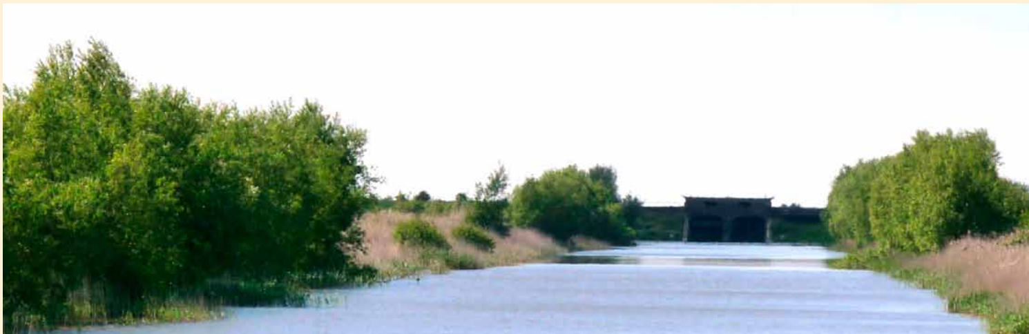
Managing water - the sluice at the end of the Huntspill River. Beyond is Bridgwater Bay and the Bristol Channel.
