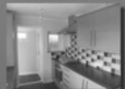
• Kitchen Installation • Tiling
