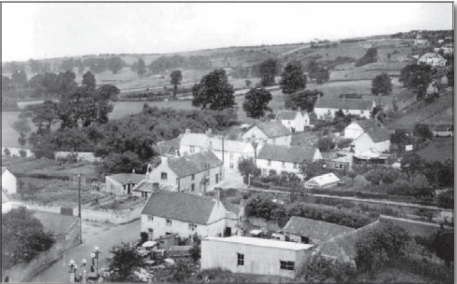
Celtic Way and Shiplate Road junction
