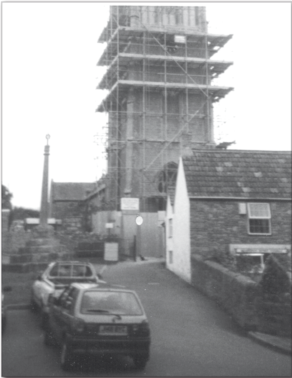
Bleadon Church with scaffolding
