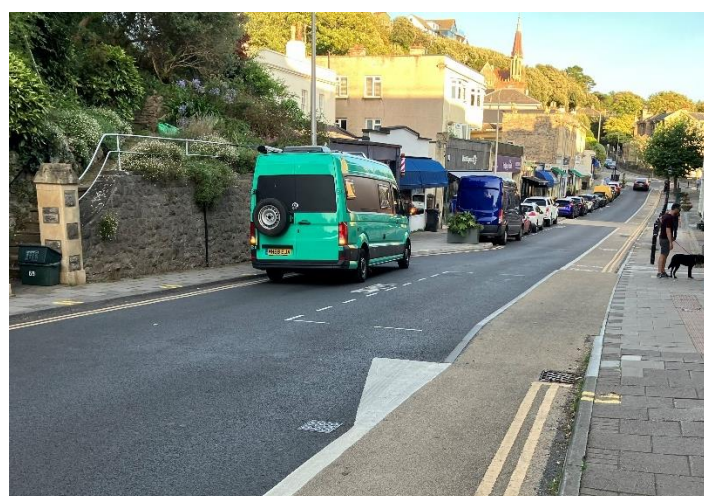
Figure 24 – Vehicle stopping outside loading bay
