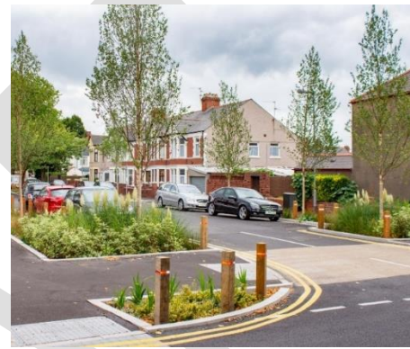
Kerbside raingardens, Cardiff
