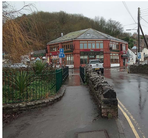
↑ Narrow footway over bridge
