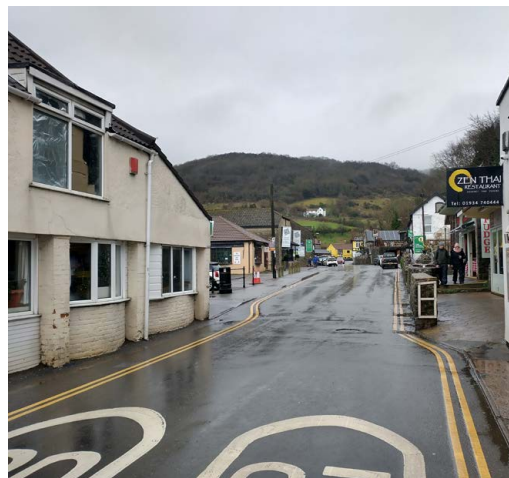
↑ Narrow thresholds with level changes
