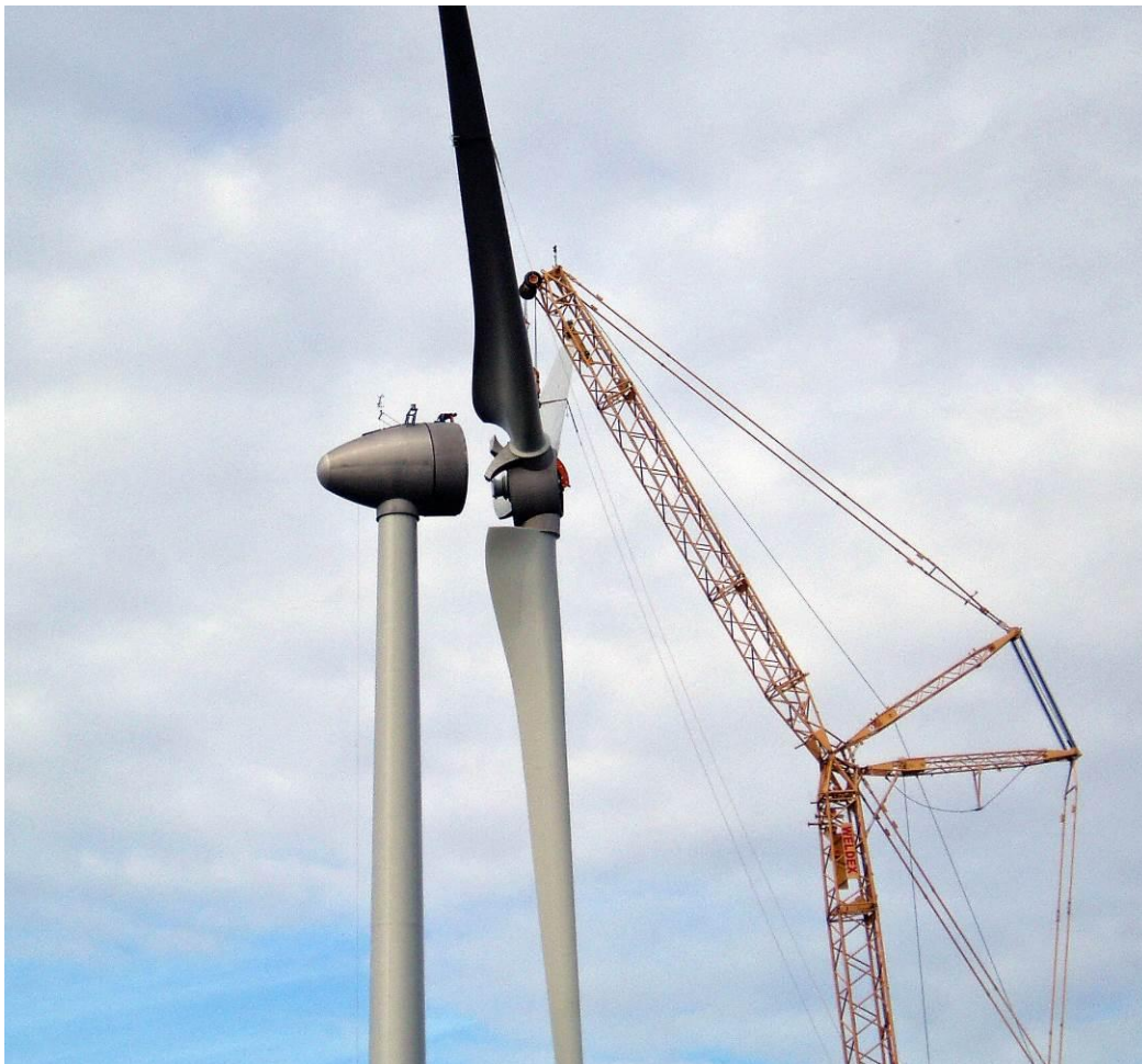
Avonmouth turbine construction. Image courtesy of Ecotricity
