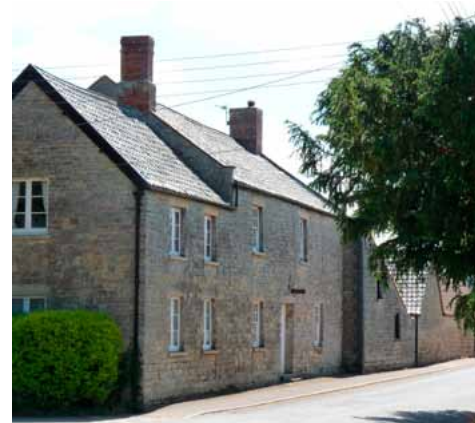
Simple vernacular architecture using local 'blue' Lias limestone in the village of Chedzoy.
